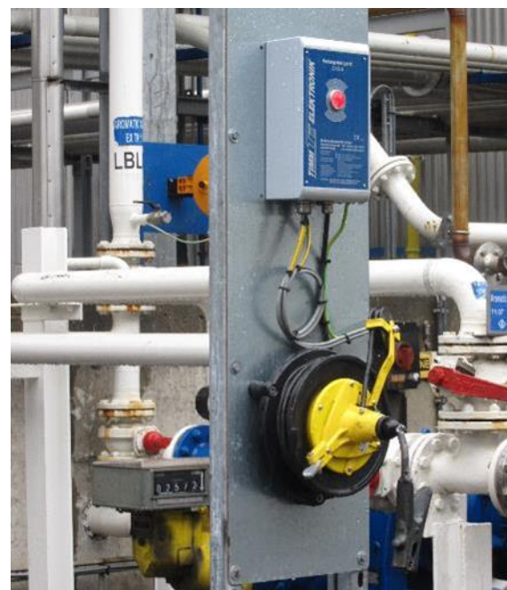
Figure 4: Installed EKX-4 with explosion-proof Cable Reel KA and Grounding Clamp EZ1
